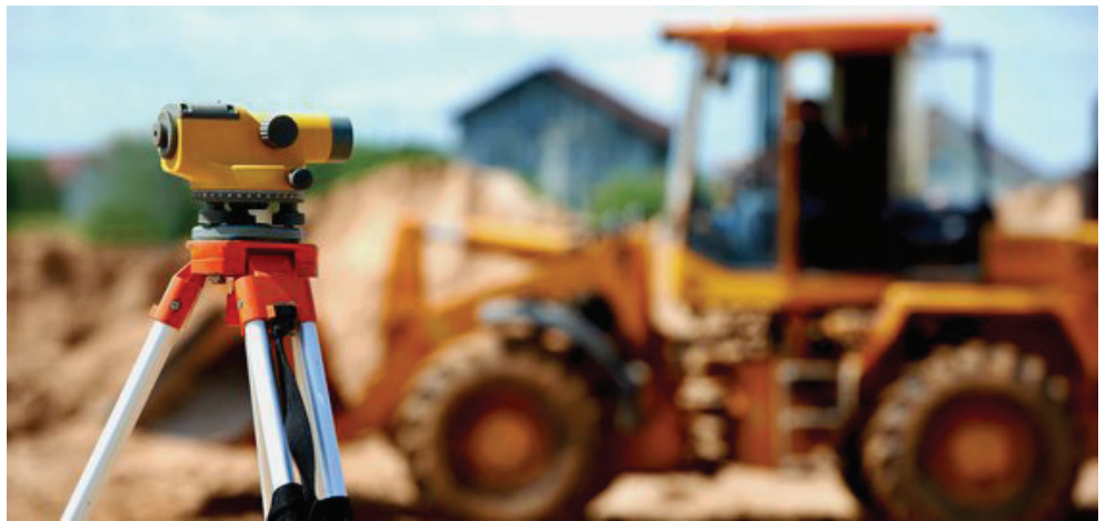
Surveying a construction site with a laser scanner
